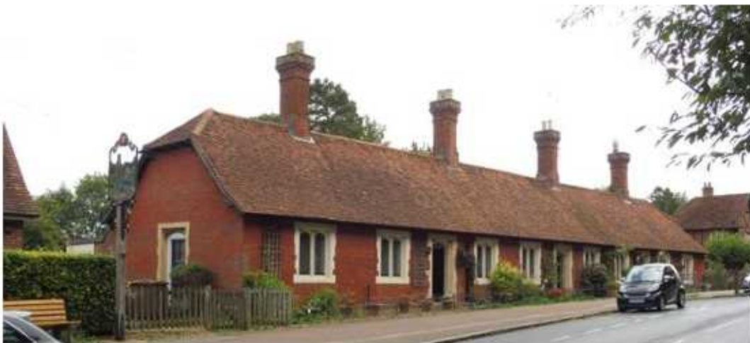
1 – 8 Tower Hill almshouses from the southeast
